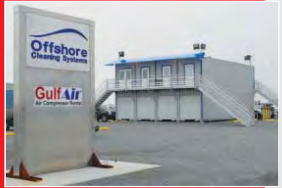
With its modular design, the Port Fourchon headquarters of Offshore Cleaning Systems can be removed completely in the face of a hurricane.
