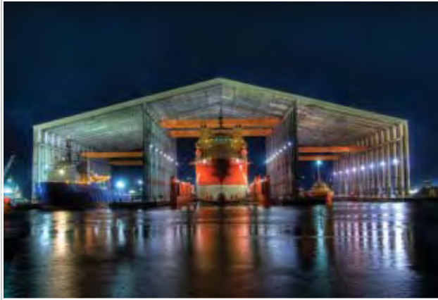
An anchor handling vessel undergoes work at the recently opened Edison Chouest covered dock in Port Fourchon.
